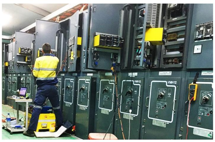
The pre-commissioning tests need to be carefully programmed so that they take place in a logical and efficient order, in order that no equipment is disturbed again during subsequent tests.
