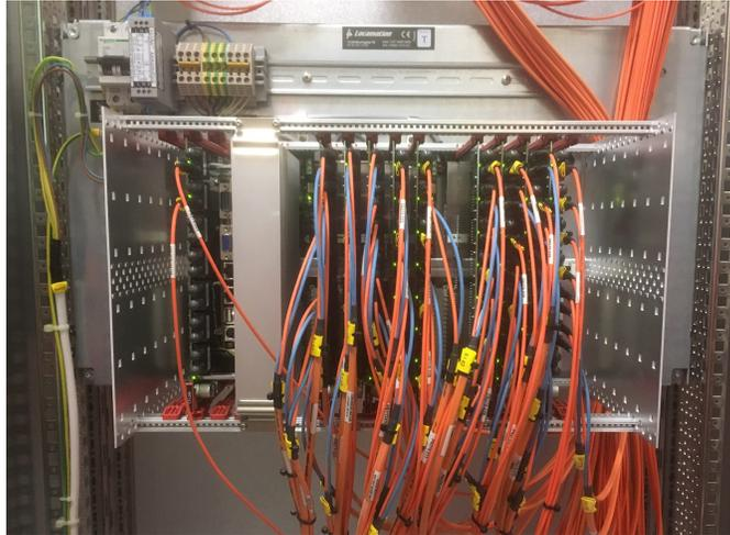
Figure 7: The Central Computing Unit installed in the substation
