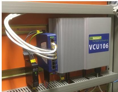
Figure 8: The Versatile Communication Unit installed in the substation
