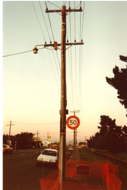
Photo 3: 11 kV Cable on Pole
