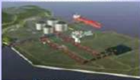
Natural gas processing
